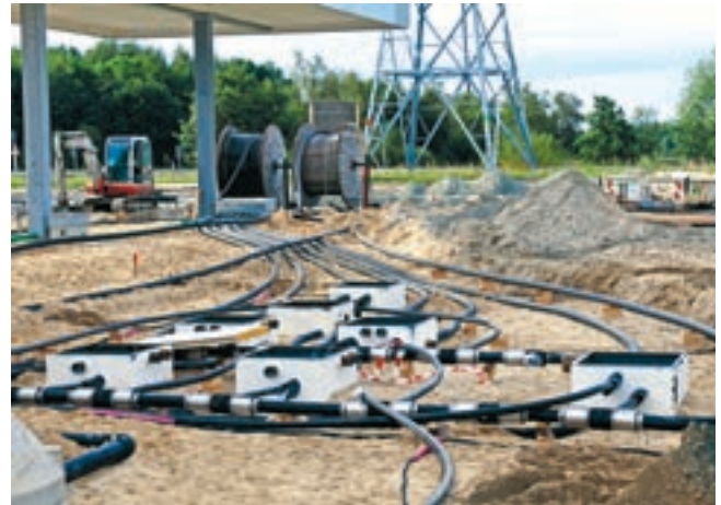
Laying the filling pipes directly off the drum
